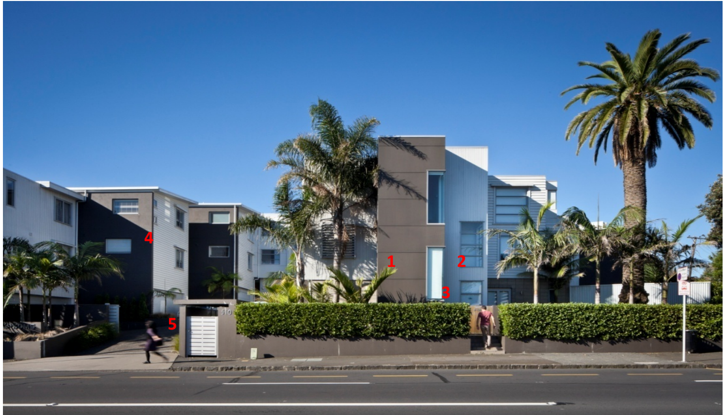
The units facing Manukau Road all have individual access from the street.
